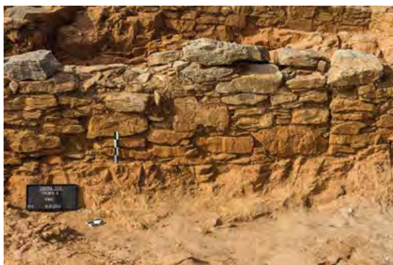
3. Detail of the stone fill of the former doorway in M1. View from SE.
